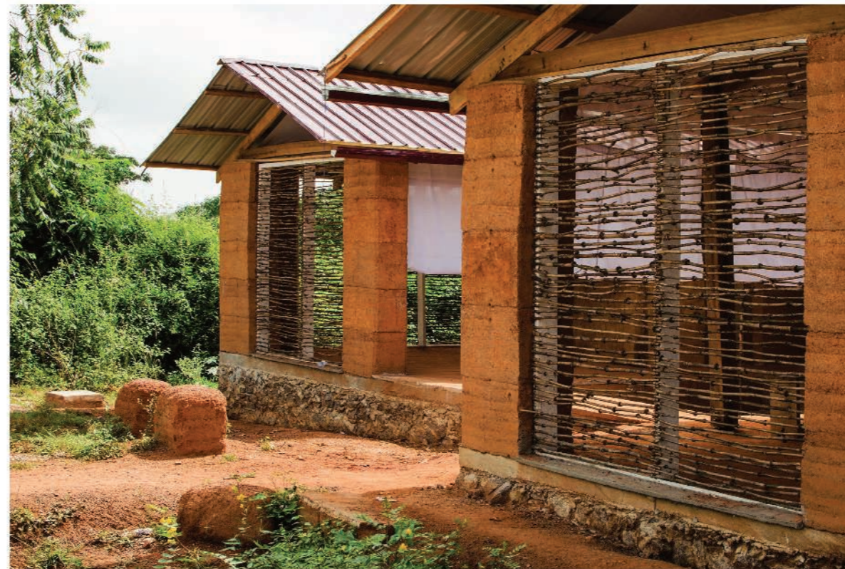
3. Finish made by Babadua canes as solar shading
